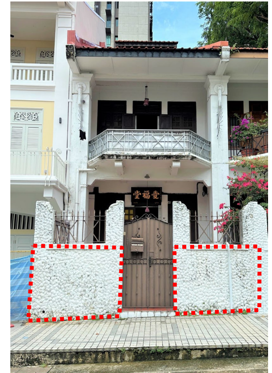
Forecourt wall with textured plaster finish
